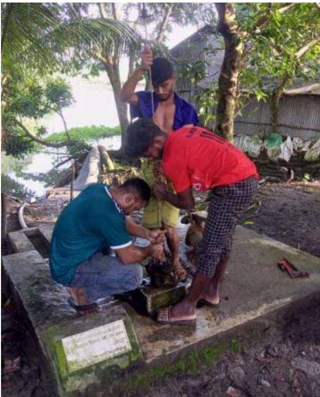
Rehabilitating water point
