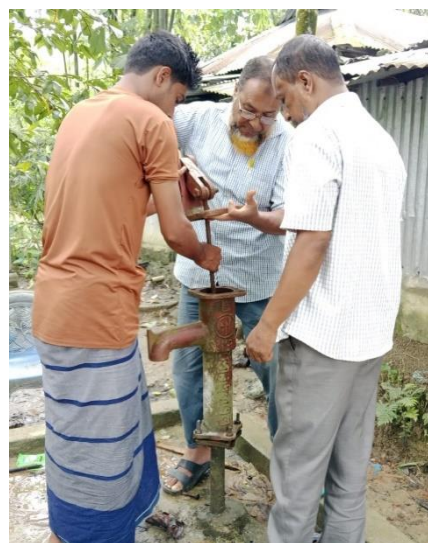
Pic-09: After rehabilitation
