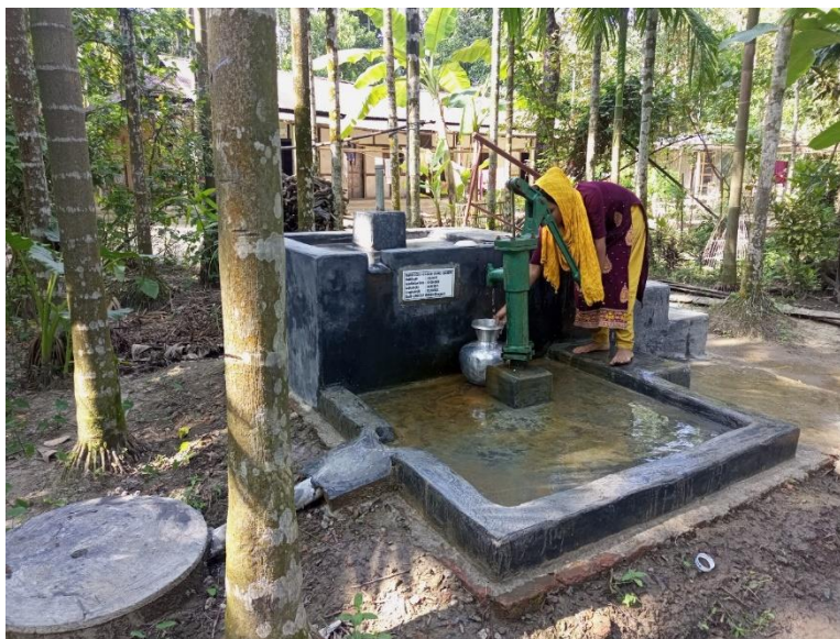
Pic:26- Raised platform during flood
