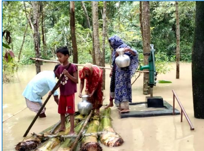
Pic:27- Raised platform during flood
