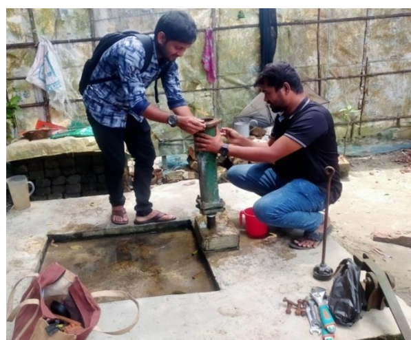
Figure 13: Rehabilitating water point
