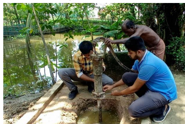
Pic-9: Rehabilitating water point
